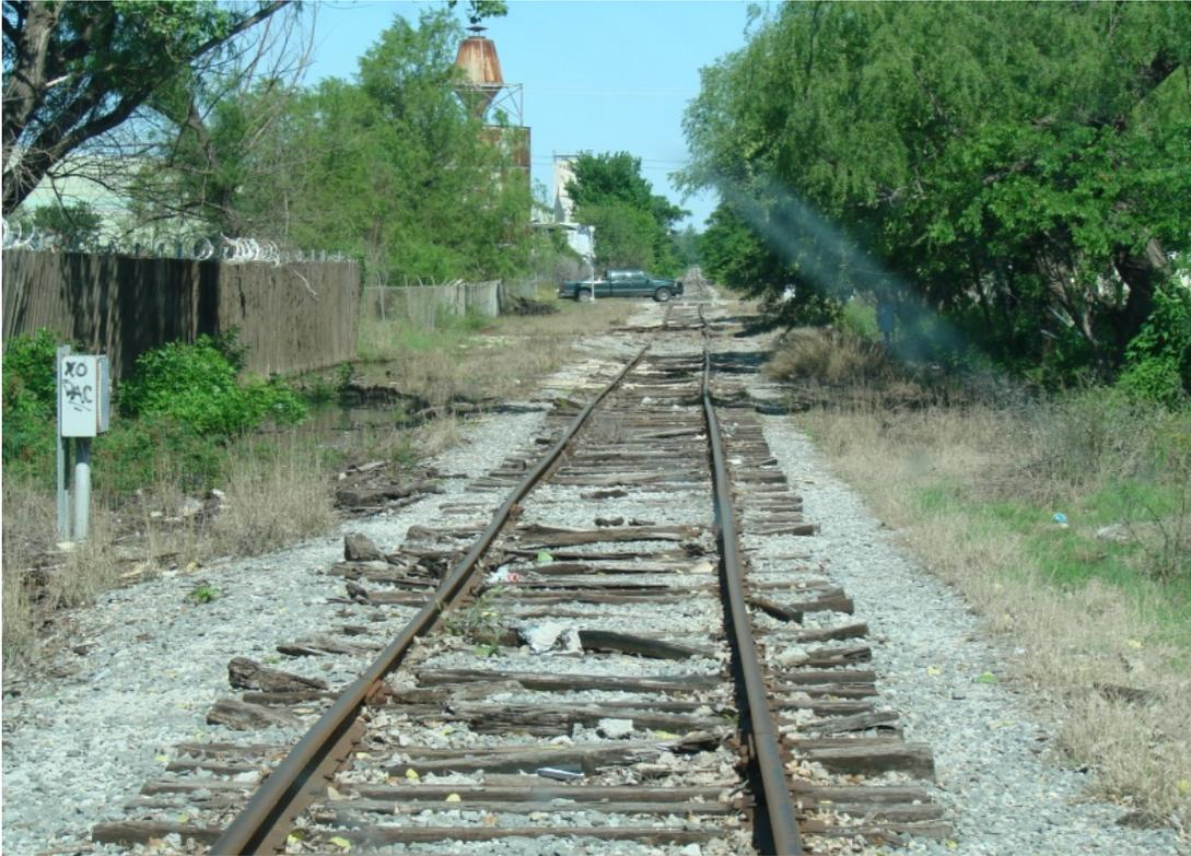
**Figure 3-15: Deferred Maintenance Prior to Abandonment**
